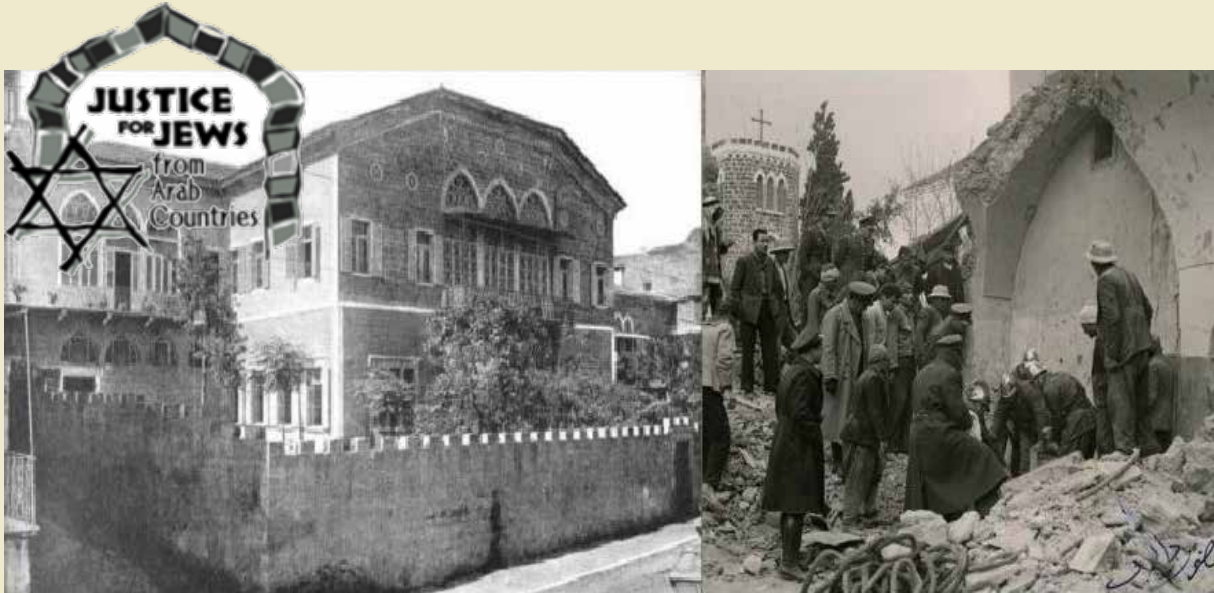
The Alliance School in Beirut, Before and After the 1950 Bombing. Source - Zafrani
