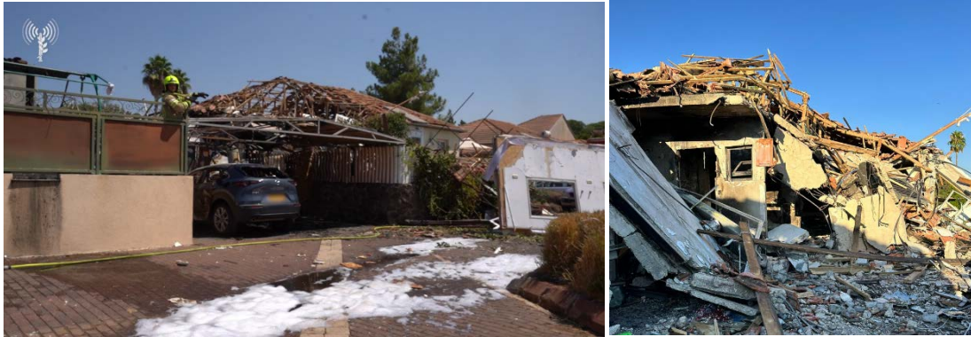
Buildings damaged in Katzrin (IDF spokesperson, August 21, 2024)
