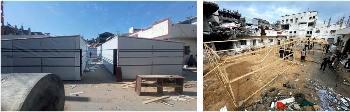
Constructing the field hospital (Kamal Adwan Hospital Facebook page, February 13–16, 2025)
