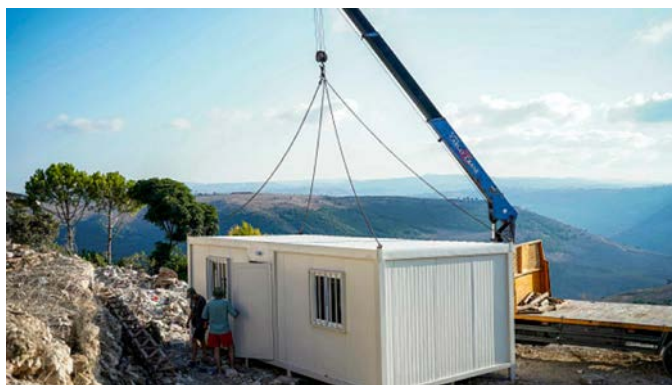
Delivery of mobile home to Zawtar al-Gharbiyeh (al-Markazia, September 23, 2026)
